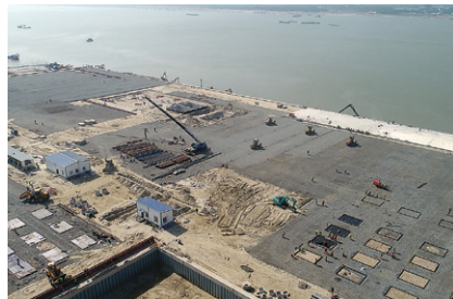
Cargo terminal at the Rooppur Nuclear Power Plant (Republic of Bangladesh)
