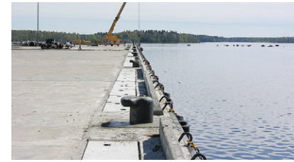
Berth #1 of the Sea Terminal of the Port of Vysotsk, Cape Putevoy
