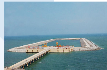
Breakwaters of the seawater intake system for cooling the first and the second generating units of the NPP Kudenkulam (Republic of India)
