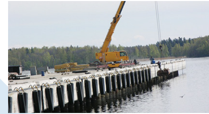
Breakwaters of the seawater intake system for cooling the first and the second generating units of the NPP Kudenkulam (Republic of India)
