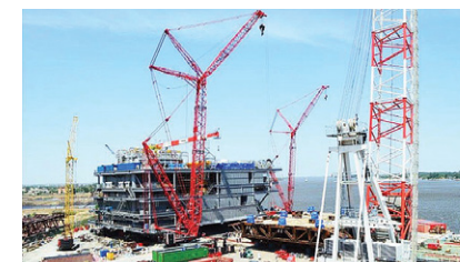
Mounting pad of marine structures at the North Caspian oil fields operated by
