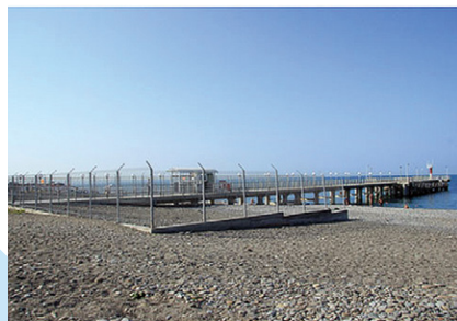
Marine passenger terminal Dagomys (a Winter Olympics 2014 project)
